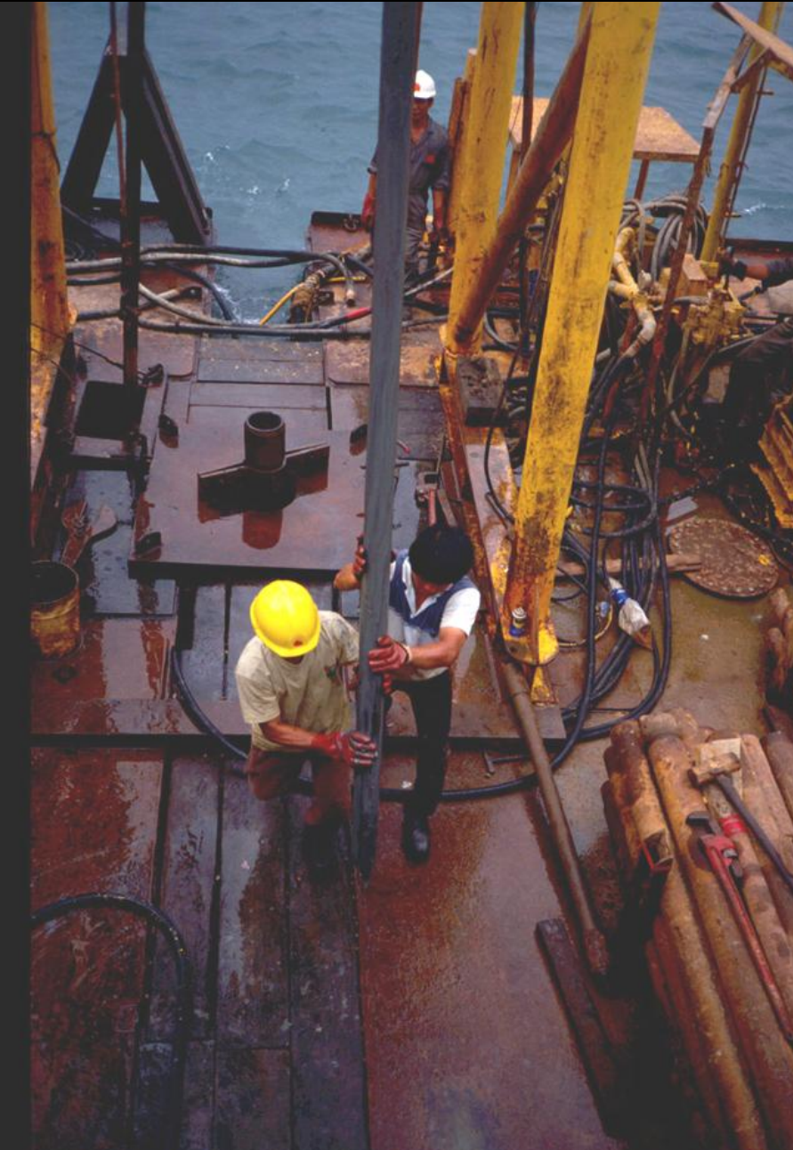
6-m drill pipe
