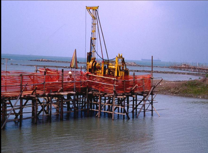
Drilling on a bamboo platform
