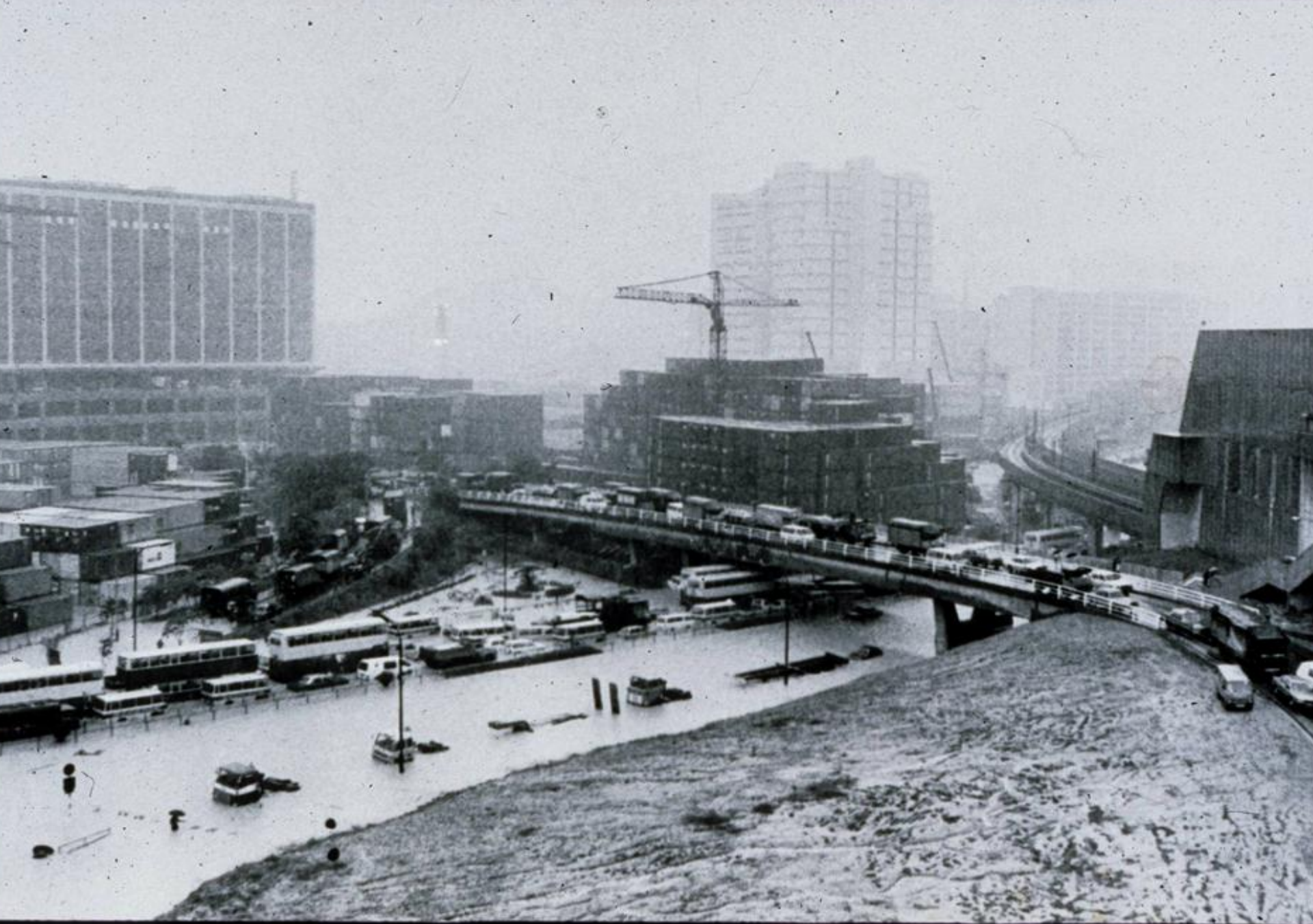
Flooding of Kwai Chung Road on August 17, 1982
